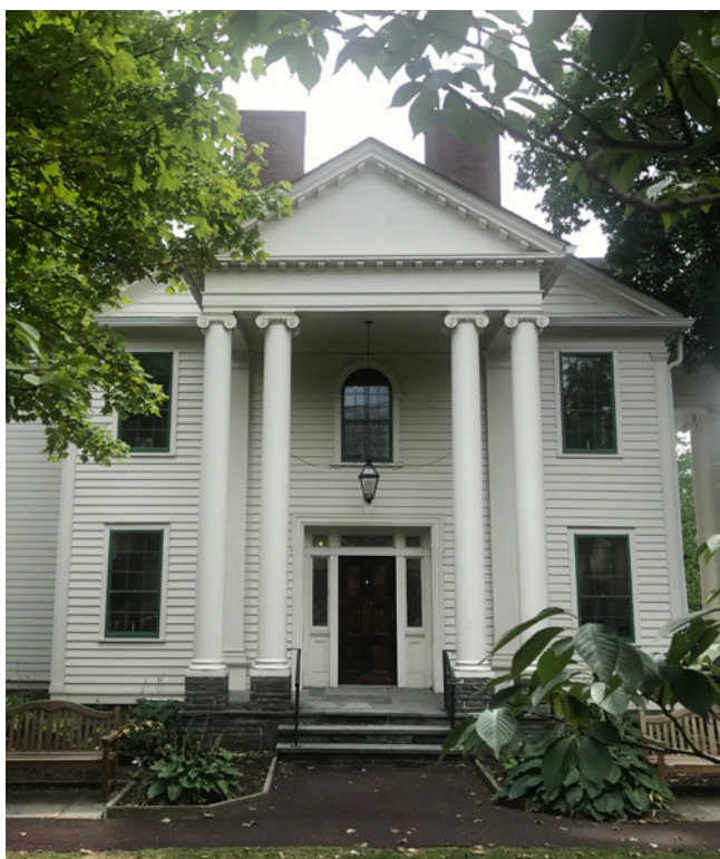
Wood siding and detailed wood pediment should be preserved.
