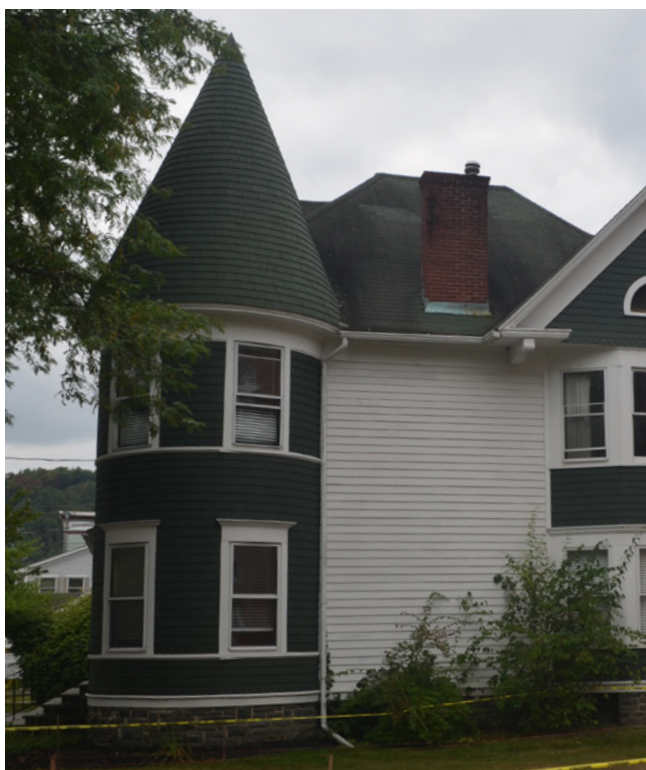
Different types of wood siding at a primary façade and secondary façades is common, like this house with singles (left) and clapboards (right).
