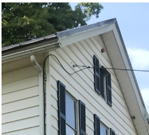
An example of a painted gutter and downspout in appropriate location to blend into the existing building.
