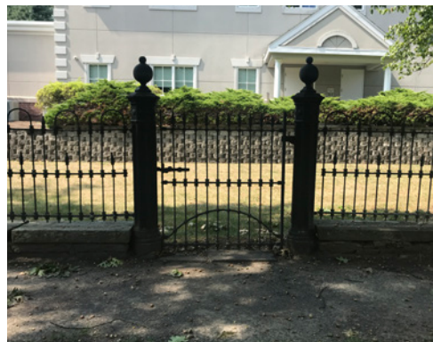
Cast iron fence with ornamented posts
