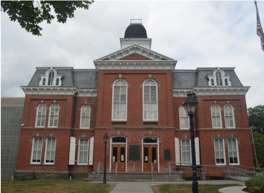
Construction of a new addition expanded the footprint of the Pike County Courthouse, which was originally designed by George Barton and built in 1874.
