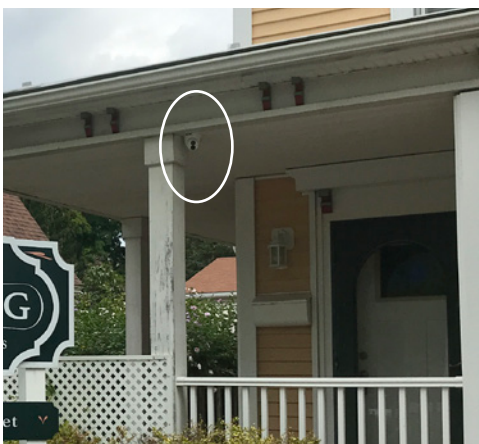
Security and communication equipment should be placed to minimize visibility. It may be unavoidable that equipment will be visible, but the immediate visual impact may be reduced through color and low profile options.
