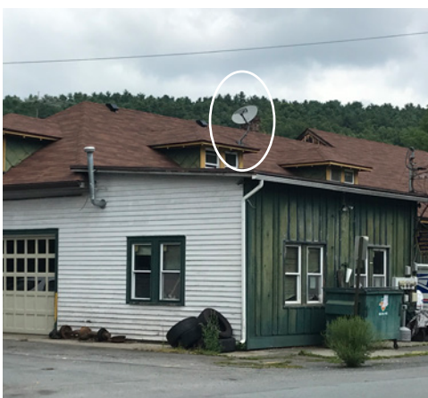
Satellites should be placed on rear roof slopes to minimize visibility from the main street. It may be unavoidable that satellites are visible between buildings on other streets, but the immediate visual impact is reduced.
