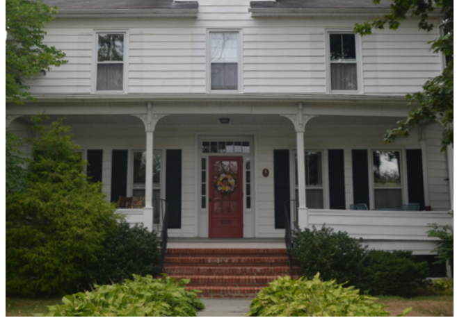
The multi-lite wood door surrounded by sidelites and a transom, and the delicate carved wood porch elements is a typical 19th century revival style entrance.
