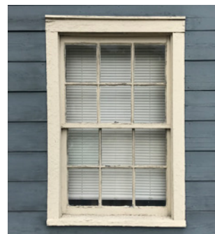
Example of a 6/6 double-hung wood window, a common historic type throughout Milford.
