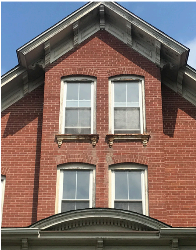
Brick masonry buildings are essential features of Milford's historic district. Details like brick segmented arches over windows should be preserved.
