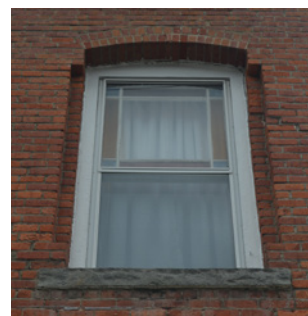
Example of a 1/1 wood window with Queen Anne style multi-color lites in the upper sash.
