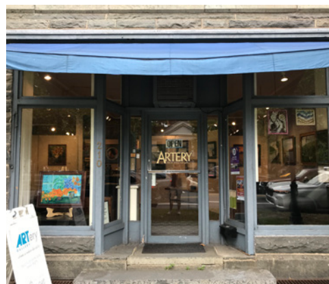
Storefronts are part of Milford's historic character, especially along Broad Street.
