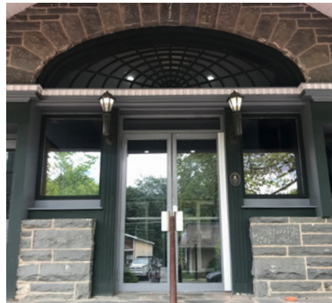
This example shows an appropriate approach for lighting replacement that mirrors the building's architectural style and its construction period.
