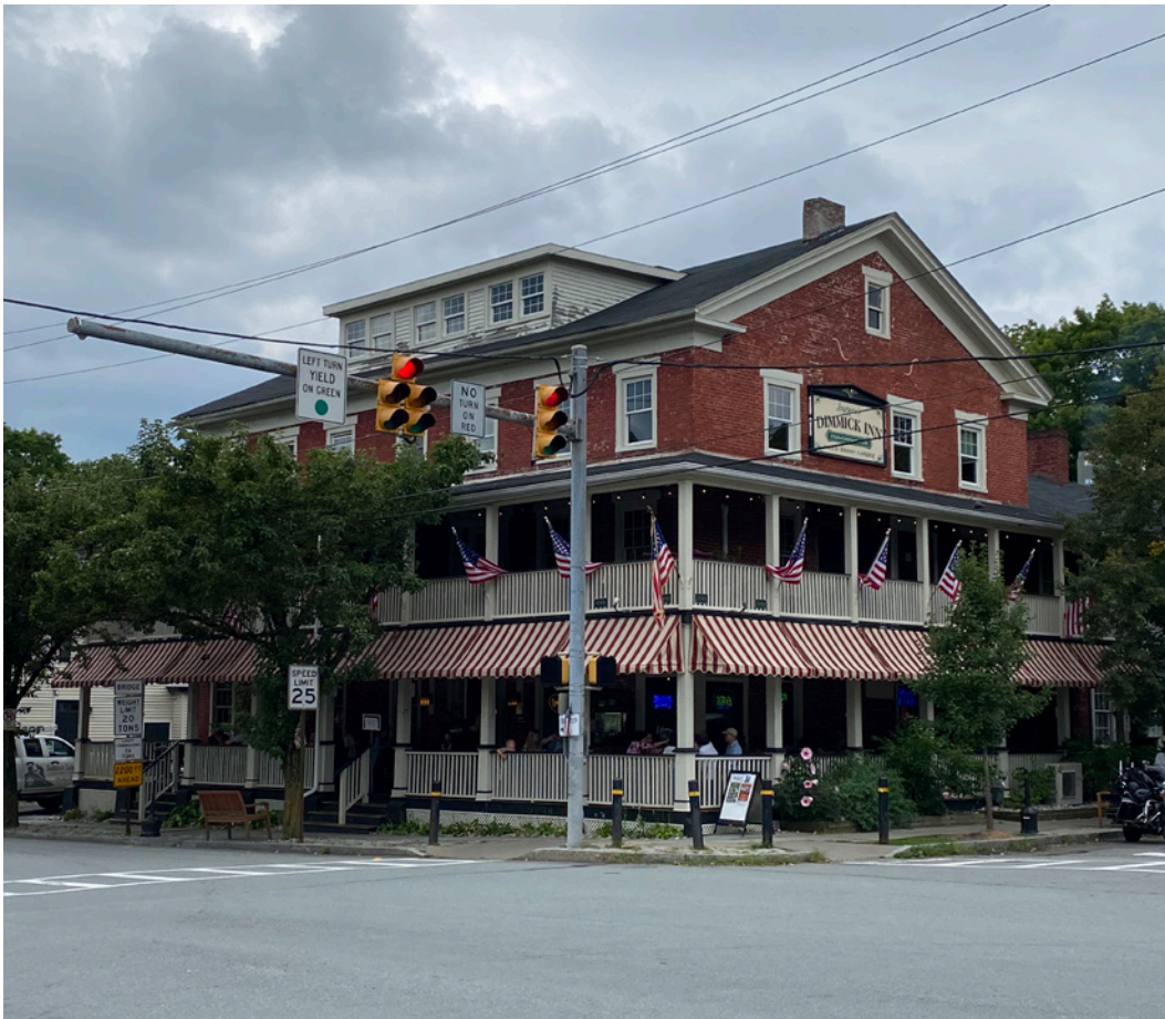
Commercial buildings contribute a great deal to the atmosphere of Milford's historic district. The Dimmick Inn remains a well-preserved commercial building anchoring the intersection of the district's two main thoroughfares.
