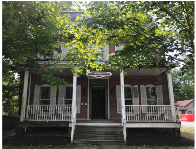
Typical historic porch components include turned wood balusters and handrails, wood steps, tongue-and-groove wood decking and ceilings, and elevated masonry foundations.
