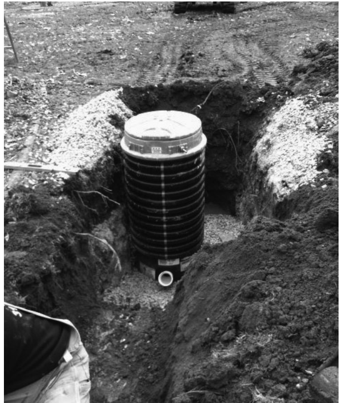
Above: Here is a view of the grinder pump system in the trench. This is prior to piping, refilling the trench with soil and leveling of the site.
